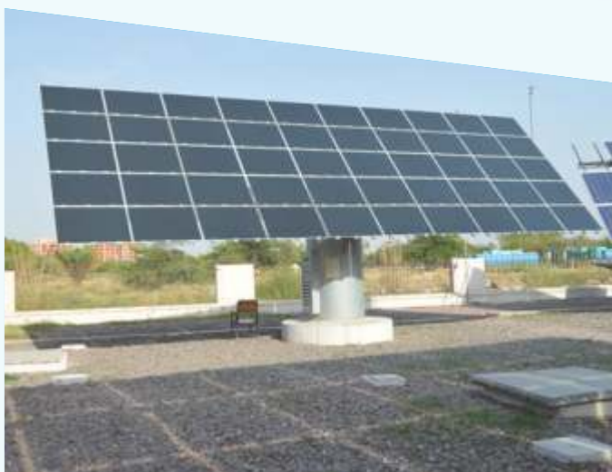
Solar Energy Research Enclave, IIT Kanpur
